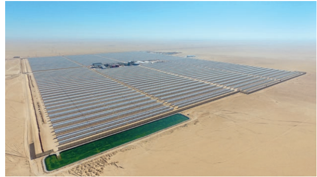
First stage of Al Sheqaya Renewable Energy Project, Kuwait. (Photo Source: GSSCPD)
